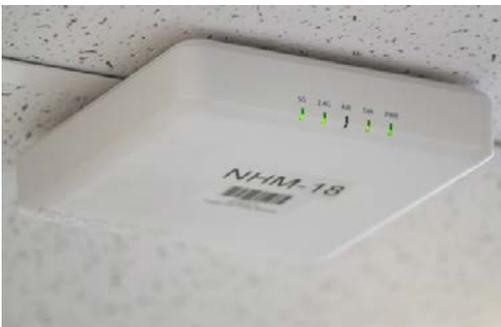
Building the wireless classroom requires reliable 802.11ac Wi-Fi to boost student achievement. The deployment consists of close to 1,000 indoor APs throughout the district. The Ruckus R500 family of APs (2x2:2 802.11ac) were deployed in the secondary schools, the H500 family of APs (wall-mounted 802.11ac) were placed in smaller areas such as offices and the R700 family of APs (4x4:4 802.11ac) were placed across the elementary schools.
