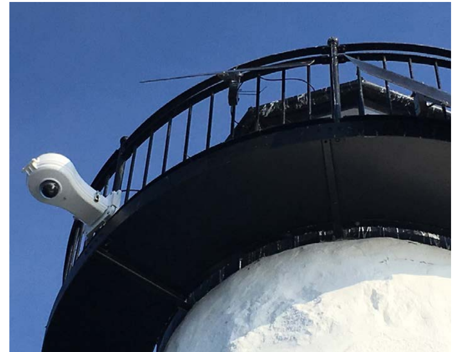
Cameras and IoT-enabled sensors on the Palmer Island Light Station increase port security data for the fish houses and help ensure boats comply with catch quotas and port regulations.
