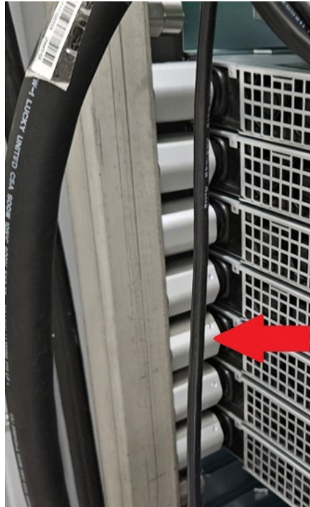
Figure 15. Direct Liquid Cooling Quick Disconnect (DLC QD) (Right)
