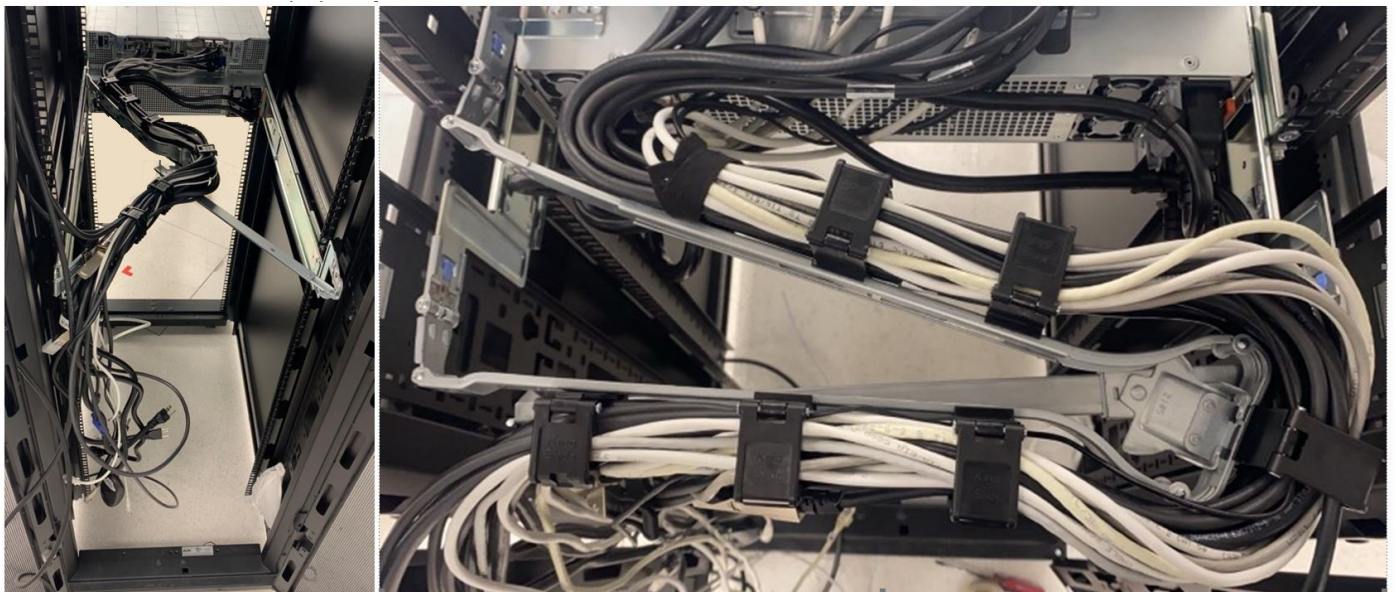
Figure 10. Stab-in Sliding rails with CMA cabling
