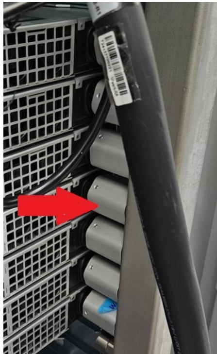
Figure 11. Direct Liquid Cooling Quick Disconnect (DLC QD) (Left)
