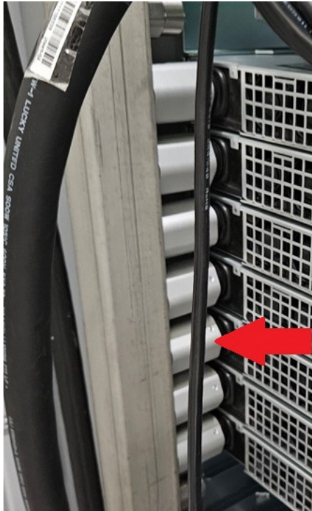
Figure 12. Direct Liquid Cooling Quick Disconnect (DLC QD) (Right)
